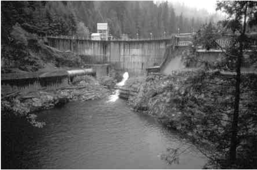
PacifiCorp's relicensing effort for its eight-dam, 185-MW North Umpqua project in Oregon—which includes the 11-MW Soda Springs Dam project shown here—is one of the U.S.'s longest running, most expensive relicensing efforts. Reform by the Federal Energy Regulatory Commission intends to make relicensings such as this one more streamlined and efficient. (Photo courtesy PacifiCorp)
